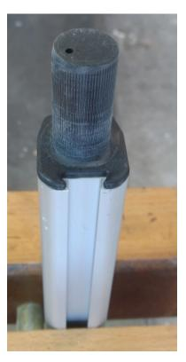
Removing the arm from the post reveals the inner bearing that is part of a larger piece of plastic that is press fitted into the post. Do not remove this.
