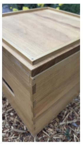
Note the detail on the half-lapped joint for the edges of the top. Yes, woodworkers would point out that this is not the proper way, since two edges run counter to the grain of the top, but the wood is reasonably stable and I have not witnessed any trouble.
